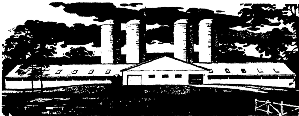
Agway free stall barn engineered for expansion
