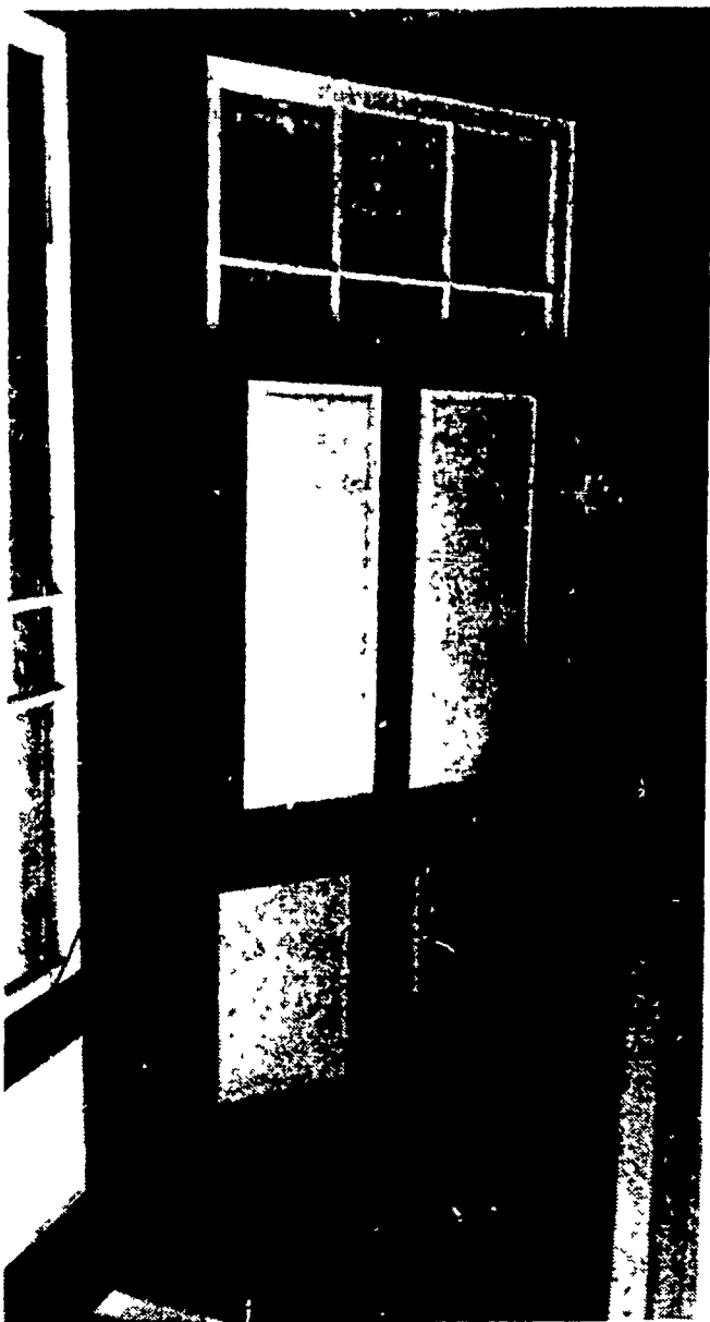
"Indian doors" were used to keep the arrows from breaking the windows in farm houses. A front panel slides up over the panes and is bolted into place as a form of protection.
