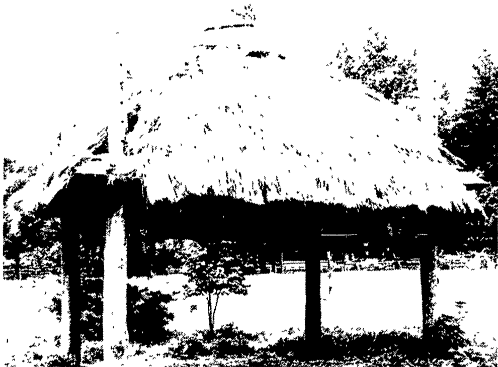
At the Settlers Village, a hay barracks was constructed to store the hay. The roof can be raised and lowered according to the amount of hay being stored.
