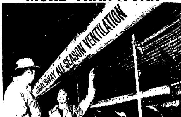
Jamesway<sub>®</sub> All-Season® Ventilation System controls condensation, odors drafts. Air intake, exhaust, and circulation are automatic.
