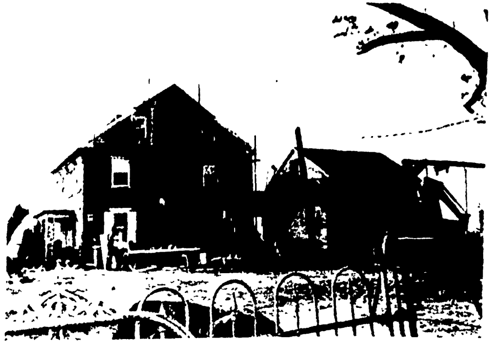
A number of neighbors and volunteers worked diligently to restore portions of the Shenk house which were torn away by the tornado.
