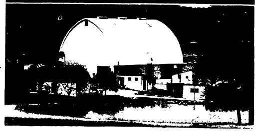
Laminated arches for barn type construction cover widths from twelve to thirty-eight feet, with heights of ten to twenty-five feet. Free Stall Housing Barns include widths of ninety feet and heights to thirty-two feet. Utility and storage buildings are available in many practical sizes.
