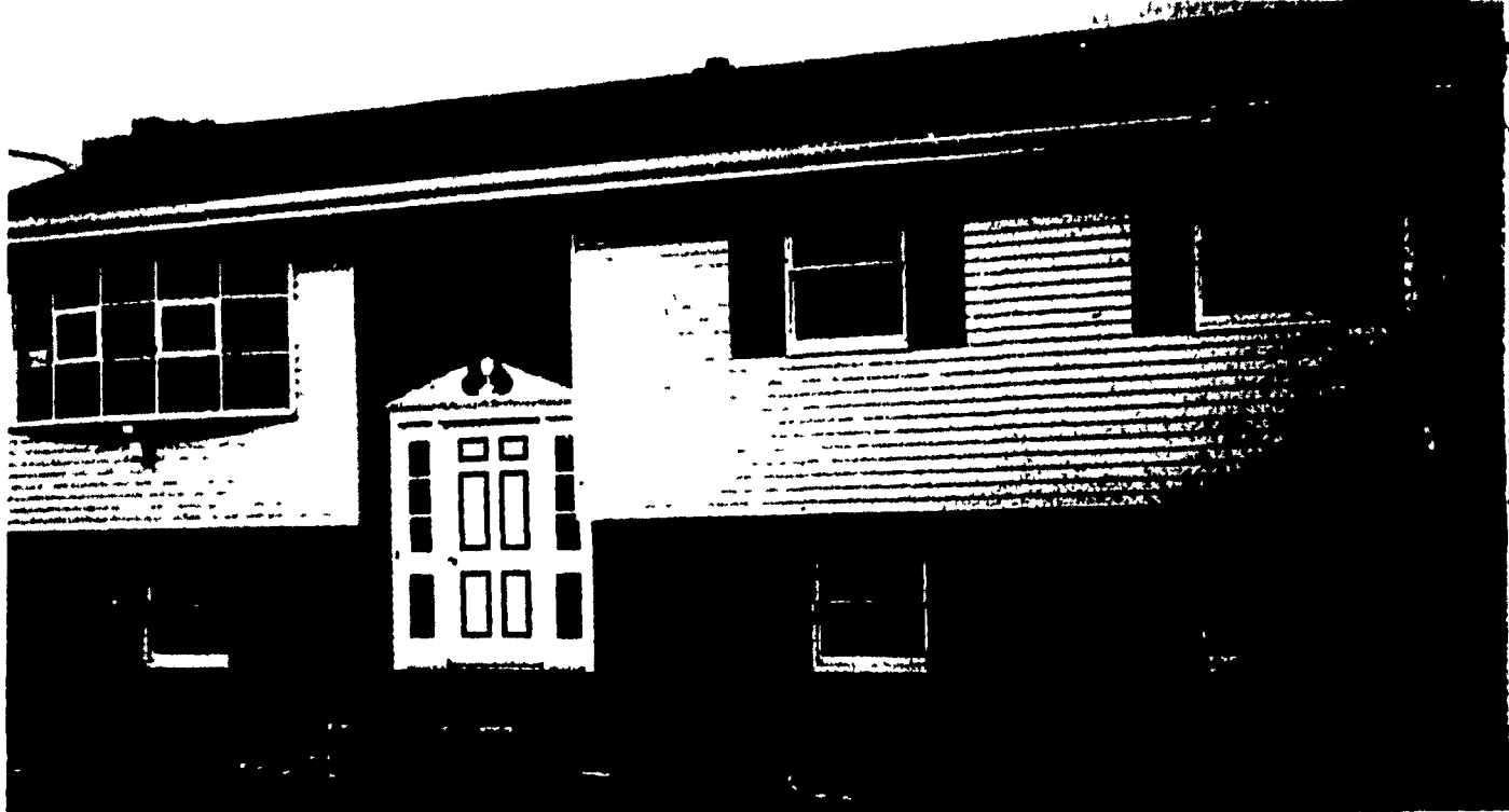
The new home of Mr. and Mrs. Thomas Enck which was built with volunteer help.
