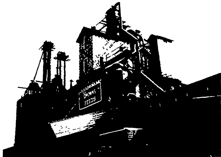
New Air-Vapor system triples bulk unloading facilities. Ingredients are delivered by either railroad or truck.
