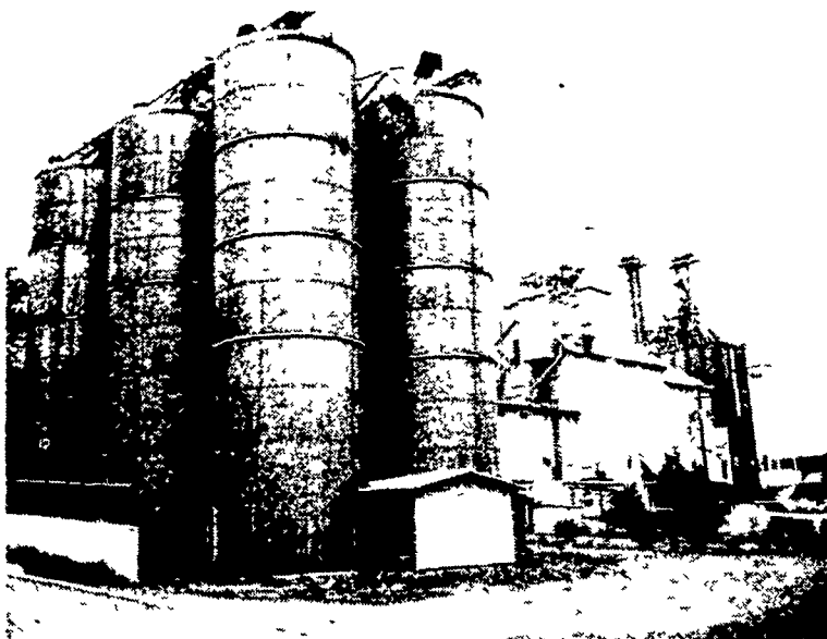
Harvester silos are used to store ingredients. Air-vapor system is used to fill and empty silos.
