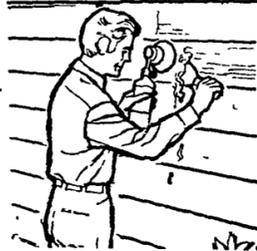
gas-fired infrared paint peeler
