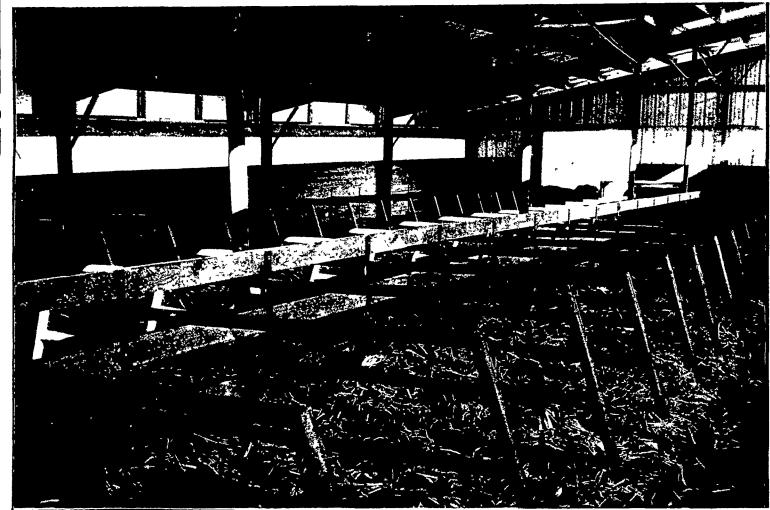
We make a high Security Free Stall from high grade boiler type steel that will last and last. A bedding board is installed and the stall is elevated above the scrape area. Extra floor space is given to each animal and a maximum drinking area is provided. A step along the feed trough allows easy access to the feed but prevents manure from falling into the trough.
