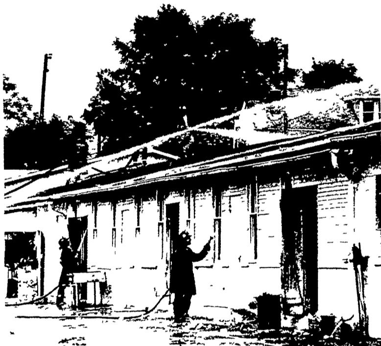
Attempts to save at least part of the main building at Root's Market and Auction failed. One fireman called it the hottest fire he'd ever experienced.
