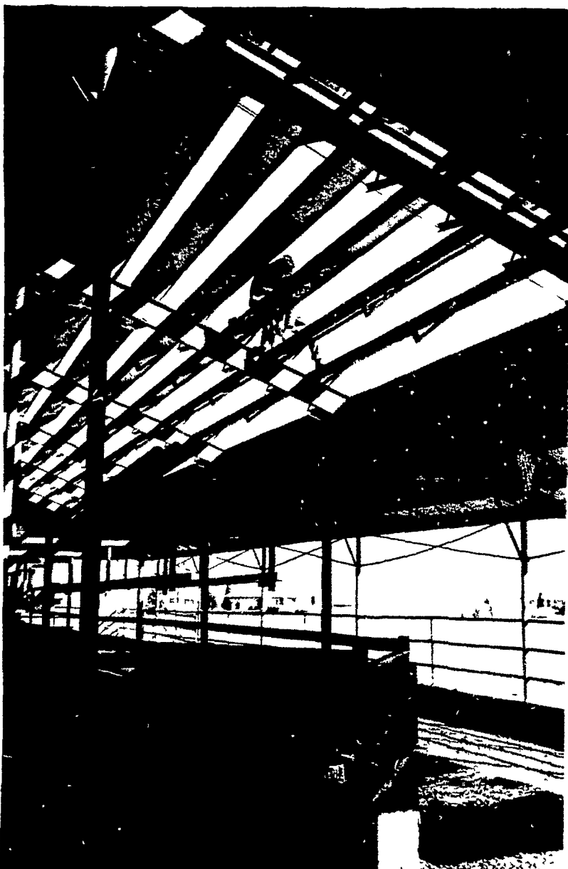
Workmen put the finishing touches on the new automatic opening and closing roof designed as part of a new livestock housing concept by Caleb M. Wenger and being completed this week at the Ernest Sauder farm at Silver Springs. The men at the top center (looking up from the ground) give an indication of the size and appearance of the new roof. These large roof panels automatically open and close, depending on whether or not the sun is shining.
