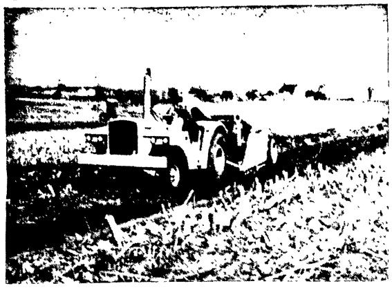
EQUIPMENT used for cut and fill method of construction. This type of equipment competes with a bulldozer as far as cost of constructing terraces is concerned.
