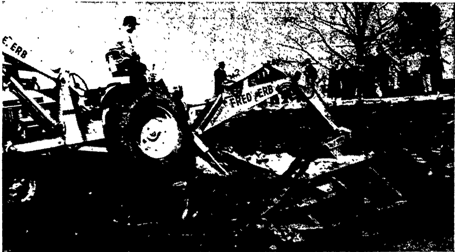
CLEANING UP AFTER A BARN FIRE at the Clarence Shultz Farm located just off Route 324 south of Marticville. The barn and livestock were destroyed
