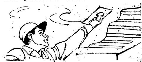
Electric ceiling cable, buried in the ceiling plaster or tiles, offers the tops in comfort and complete freedom in placement of furniture and draperies.
