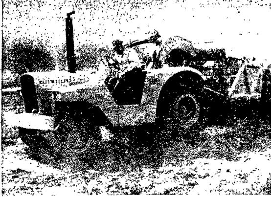
ONE OF THE RIGS used to shape waterways is this self-loading pan pulled by the tractor shown here on the Jonas and David Nolt farm near Wakefield Orval Bass, SCS county conservationist, explained that as the pan is pulled along, a cradle not feed on everything that slaushter, breaks up the dirt in a dish shape, and paddles load it into the pan A bulldozer may also be used effectively for this work. Bass noted L. F Photo
