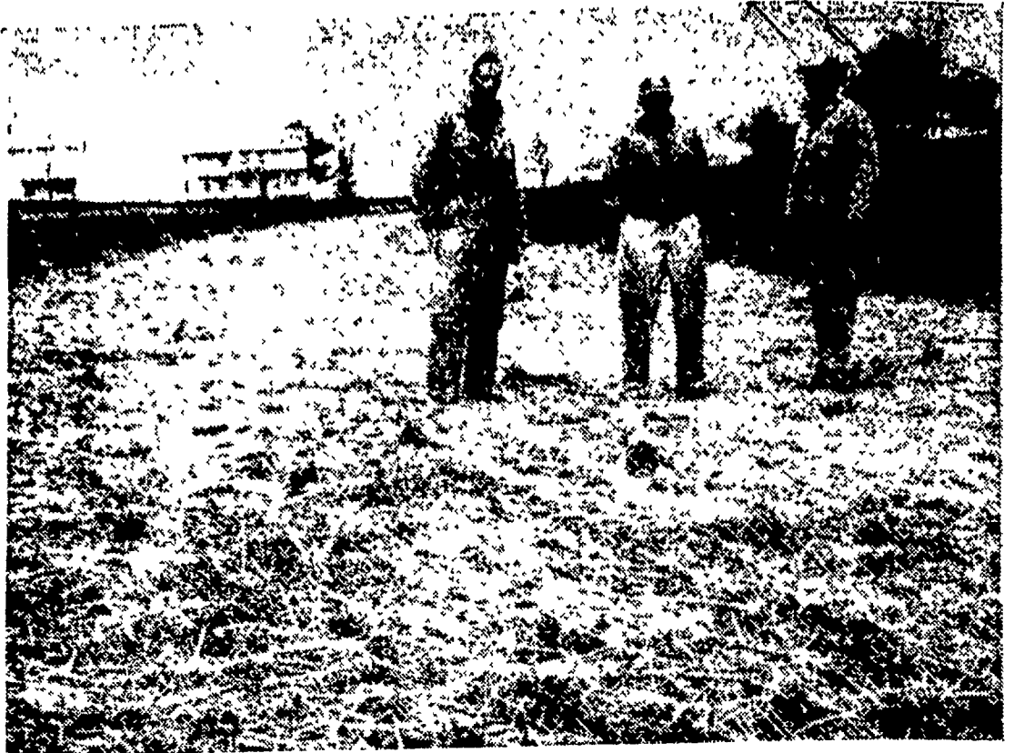
PART OF THE 6000 feet of waterways on the Neff farm at Millersville R1. From left, Robert, Christ, and Richard Neff shown on this newly constructed waterway give the viewer an idea of the width and contour of this conservation device. L. F. Photo
