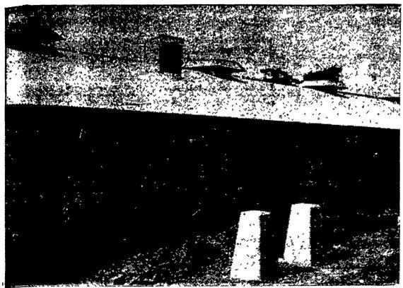
THIS SHOT OF HOUSE 1 shows hooded vents for ceiling fans and louvered vent for special attic space fan which comes on when temperature in attic reaches 90 degrees. At bottom center, exit for manure auger may be seen. Auger pipe, on the ground behind piling, will elevate manure at about a 25 degree angle into a waiting manure spreader. L. F. Photo
