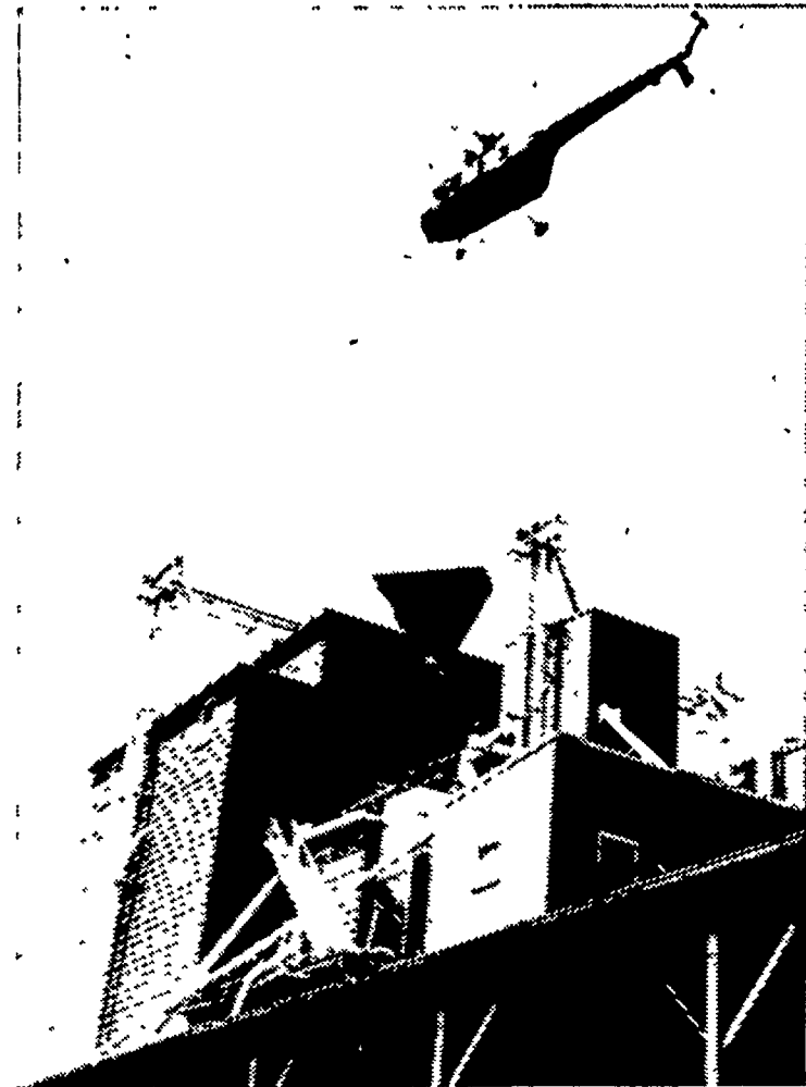
OPERATION SKYHOOK — Helicopter hovers over roof of Red Rose feed mill at York, slowly lowering bin hopper into position. The copter took part in positioning six bins as part of a $68,000 construction program to increase finished feed storage capacity at the York plant.
