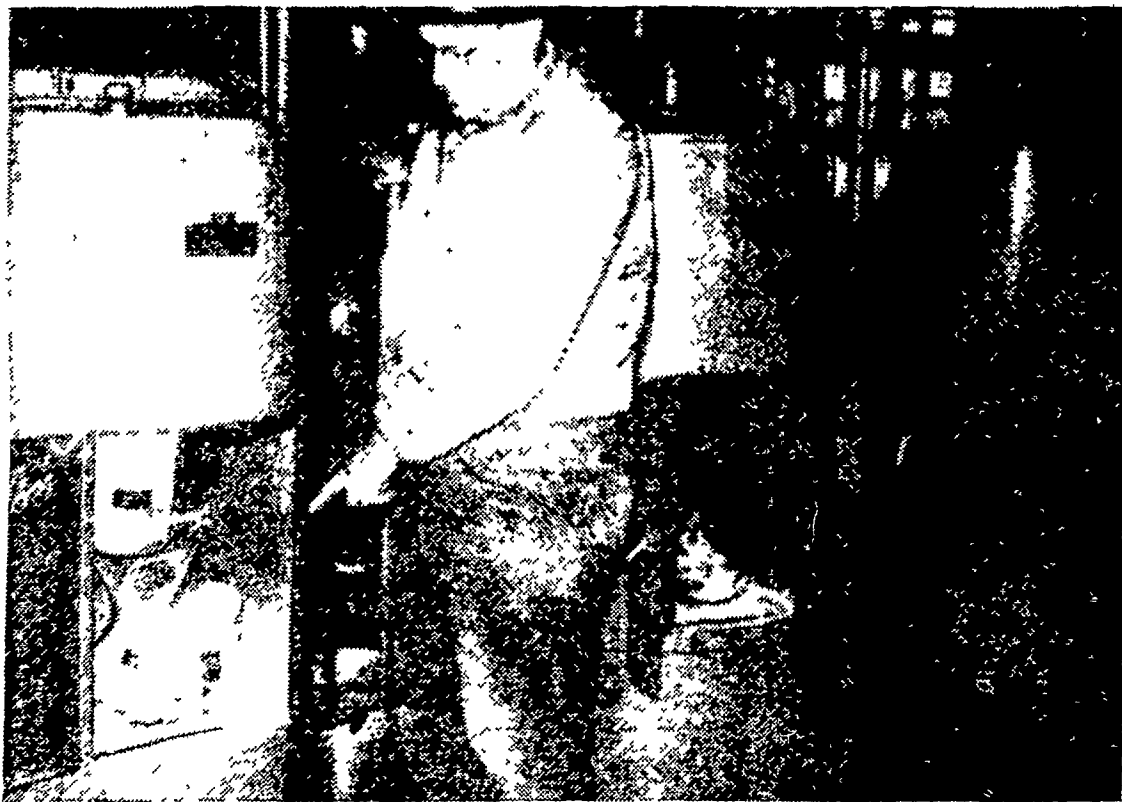
JAMES H. RUNYON OF GRACE MINE points out how chemicals are metered into pond water as part of the process which purifies the potable water supply for the plant. The other two metering devices behind Runyon are for alum and carbon.
