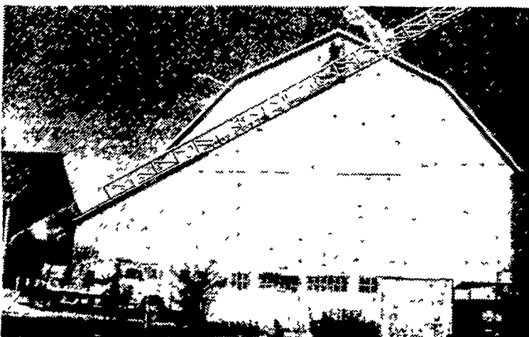
Aerial Ladder Equipment Used To Paint Your Farm Buildings
