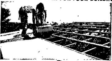
Nails tight. Self-sealing. "Just roll it on and nail it down," Galvanized steel ... or baked-on colors.
