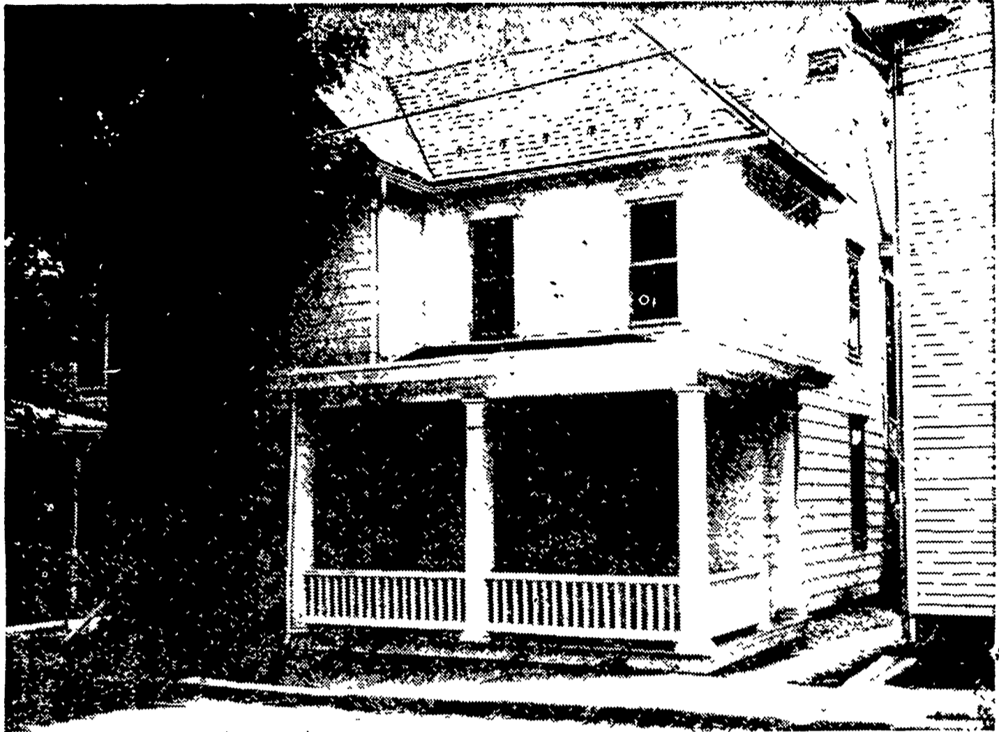
Mr. and Mrs. Glenn Badorf's all-electric home at 207 N. Cedar Street, Lititz.
