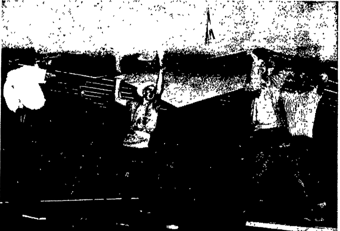
Low-cost, plastic-coated structural material developed by Container Corporation of America can save 1/3 the cost of installing combinations of conventional materials. Now being used commercially in the construction of agricultural buildings, Concora-Ply is easier and more quickly installed and therefore cuts labor costs. It can be sawed, nailed, drilled, and sanded, and is workable with standard wood-working tools. Concora-Ply was developed by CCA's Research and Development Center, Oaks, Pa. Call Kuipers Bros., New Holland 354-5146 for the name of your nearest franchised dealer. —Adv.
