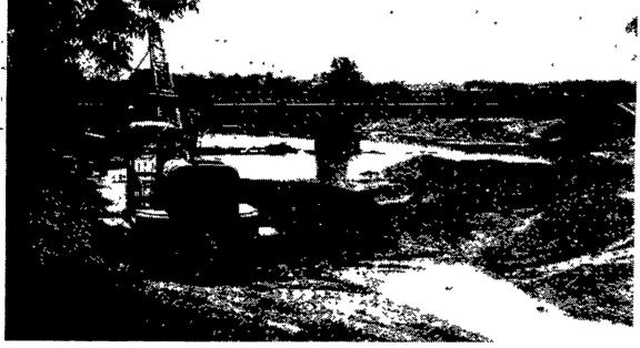
WHAT APPEARS TO BE A GIGANTIC MINING OPERATION is in reality a silt removal project under Becker's Bridge over Little Chickies Creek. Over 17,000 cubic yards of silt and sand had to be removed from the stream channel to let flood waters move under the bridge. Silt had changed the channel to the point where the bridge foundations were being threatened.
