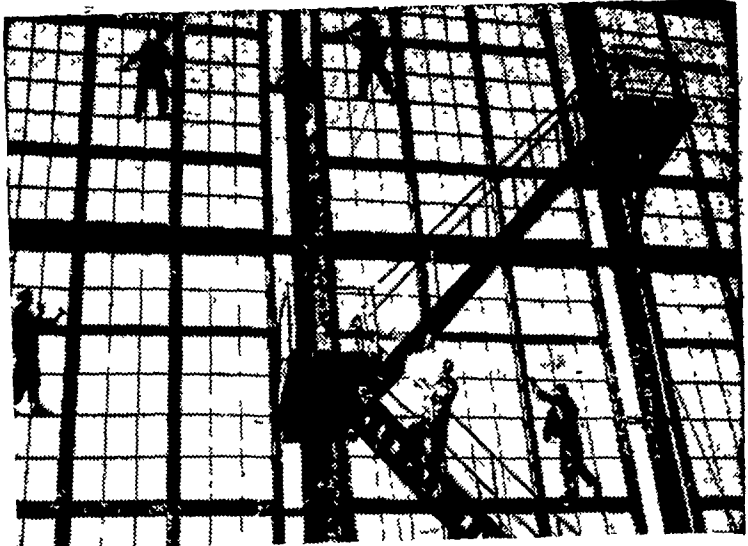
POWER PATTERN . . . Russian workmen erect a modernistic framework for a new open-hearth furnace steel mill being constructed somewhere in the Urals.
