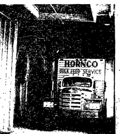
Eight 20-ton bulk holding bins at the Hornco mill make it possible to give faster service by loading a 12 ton bulk truck in 8 minutes.
