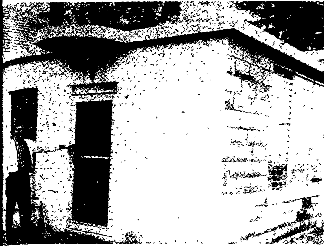
CONSTRUCTION ON THE NEW SALES ROOM at Spruce Villa Farm, Lititz R1, is most complete. Neil Clark, at the door to the sales room, hopes to begin selling milk in gallon lots at the farm early next week. Milk will be sold at wholesale prices at the farm, but it must be sold in the consumer's container. All milk at Spruce Villa will be sold pasteurized and homogenized. —L F Photo
