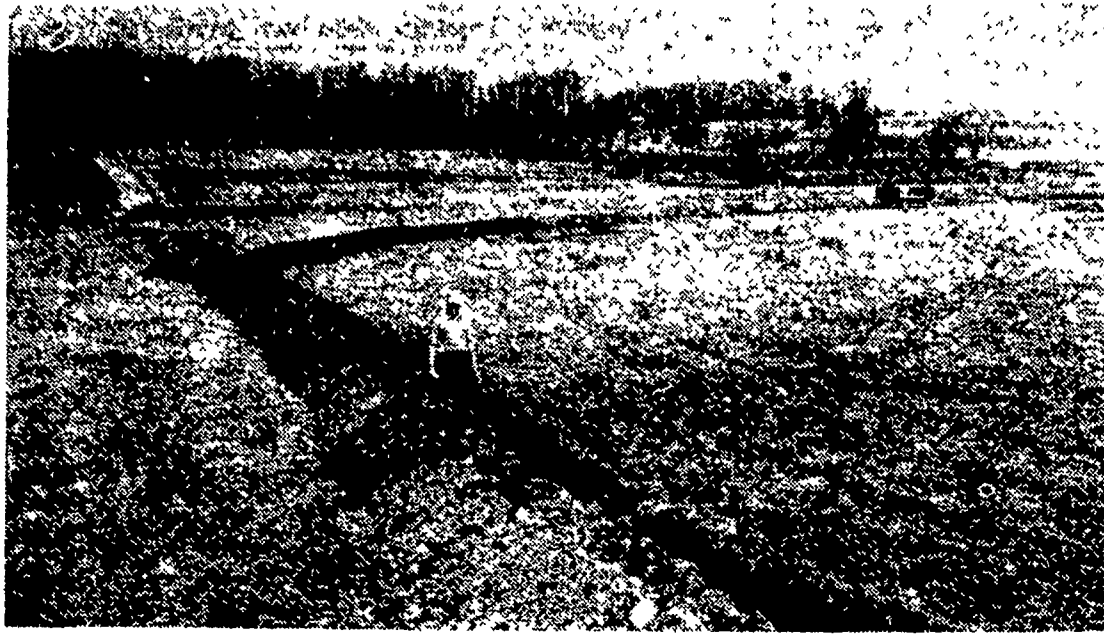
KEIFFER IS SHOWN standing by the central 6-inch tile line just above the lower laterals in the field. Above him on the hillside five laterals had been completed, while the machine was moving in to work in the "wet" lower section of the field. The part of the field below the wagon and truck has been used for pasture and meadow in the six years Kieffer has operated the farm, being too wet to crop. He hopes to start cropping it in 1960 —LG PHOTO
