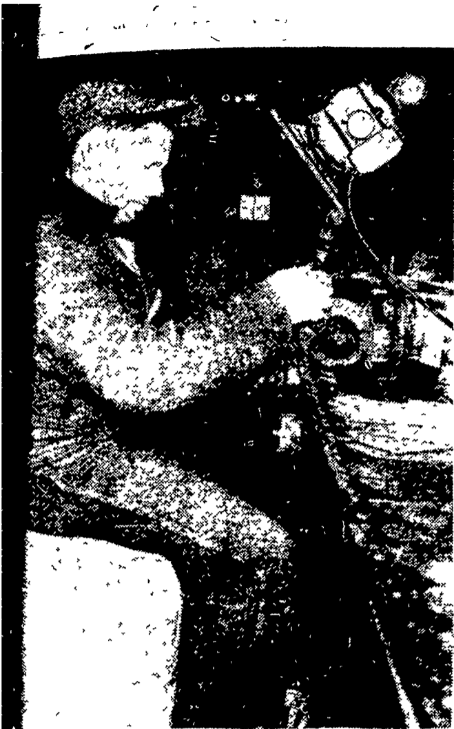
OFF SPENDS odd winter time at repair jobs, such as opening mower knives on his "lazy-man's" grinder. A long angle-iron support the knife and the powder-wings into position from above —LF PHOTO
