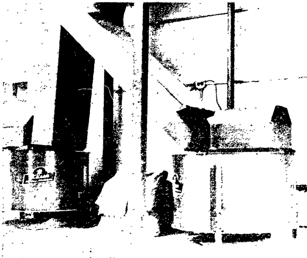
THE CHUTES coming through the ceiling, gravity feed mash and pellets from one of the five-ton capacity roof-top bulk feed bins on the house. Feed drops directly into
