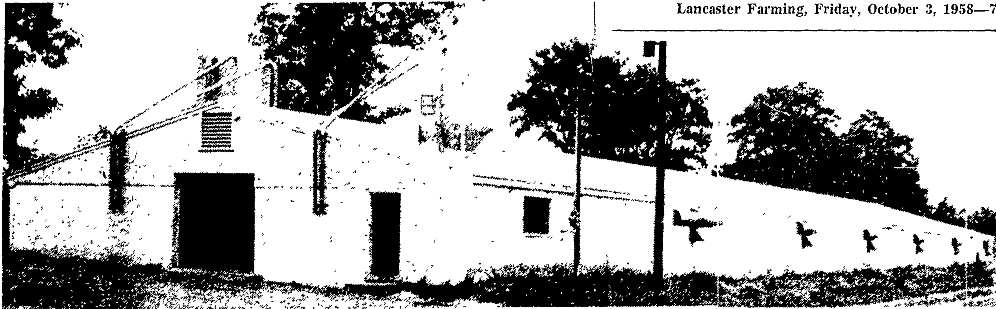
THIS OUTSIDE view of the 216-foot-long windowless house, shows its compact construction, the service doors, air vents and bulk feed bins
