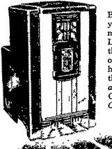
Behind the gleaming, porcelain cabinet, you'll find a patented unner unit that makes traveling floor heat possible. Look at the big, furnace-type blower that drives the air through a battery of unner heat tubes that set right in the heart of the fire! Siegler doesn't wait for the heat to come out ... it goes right in after ut, then forces it over your floors! Come in and see for yourself why Siegler Outheats-outlasts all others!
