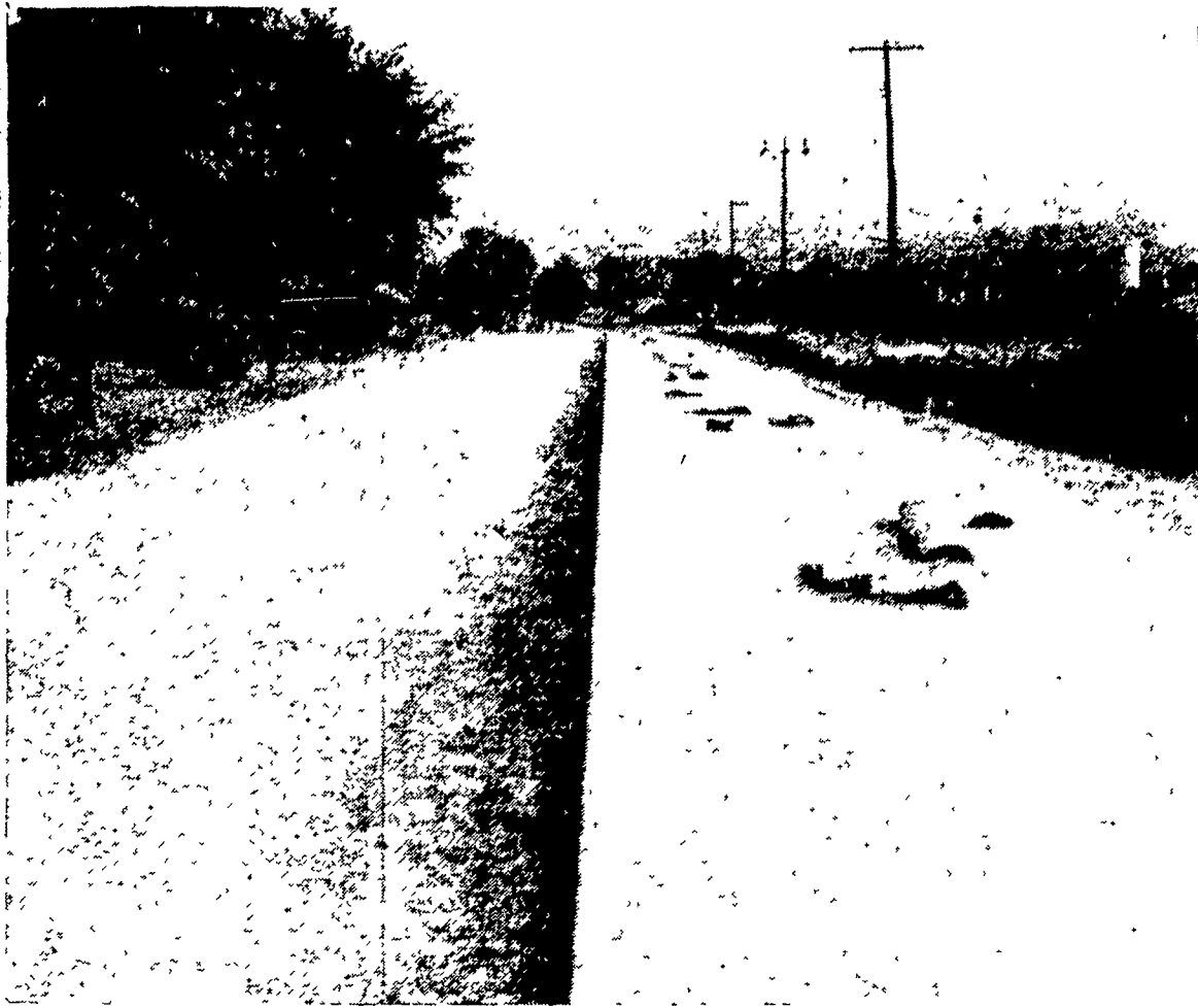
SOUTHERN LANCASTER COUNTY residents who depend on Route 222 for travel to Lancaster are happy to see concrete being laid on the sections now closed to traffic. The highway has been closed since early this spring after having been open for only a few months. The work this year will straighten some curves and will by-pass Refton. (LF Photo)
