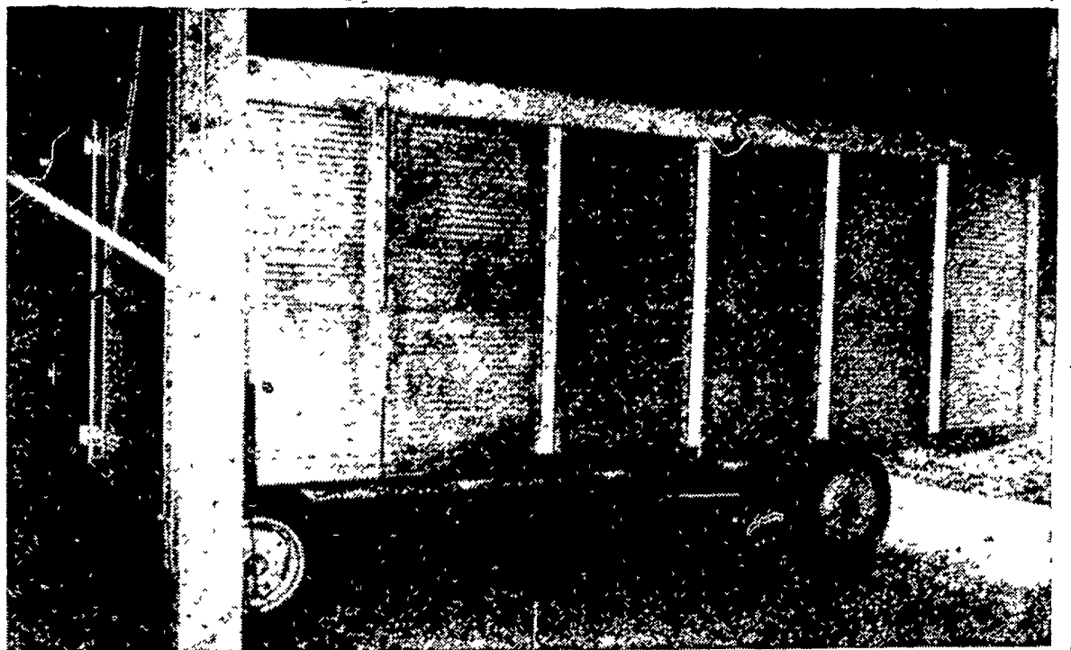
arrangement used to direct heated air from the overhead duct into the drying wagons. The lever at the left is used to
