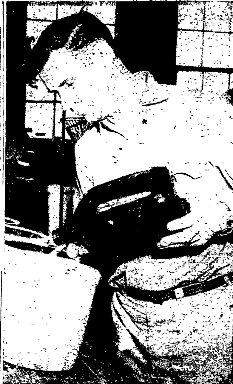
(right) HERE IS THE FIRST step in the treatment of tobacco seed against wildfire. John Jacob Oberholtzer, R1 Bird in Hand, adds a 1:1000 solution of silver nitrate to the cleaned bagged seed. Note that a common earthenware crock is used to soak the seed. The seed is soaked for 15 minutes
