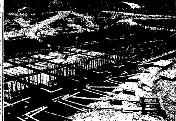
With completion of two more settling basins and four filters at the Pine Grove filtration plant, the City of Chester will draw 30 million gallons of processed water a day from the Octoraro Creek instead
