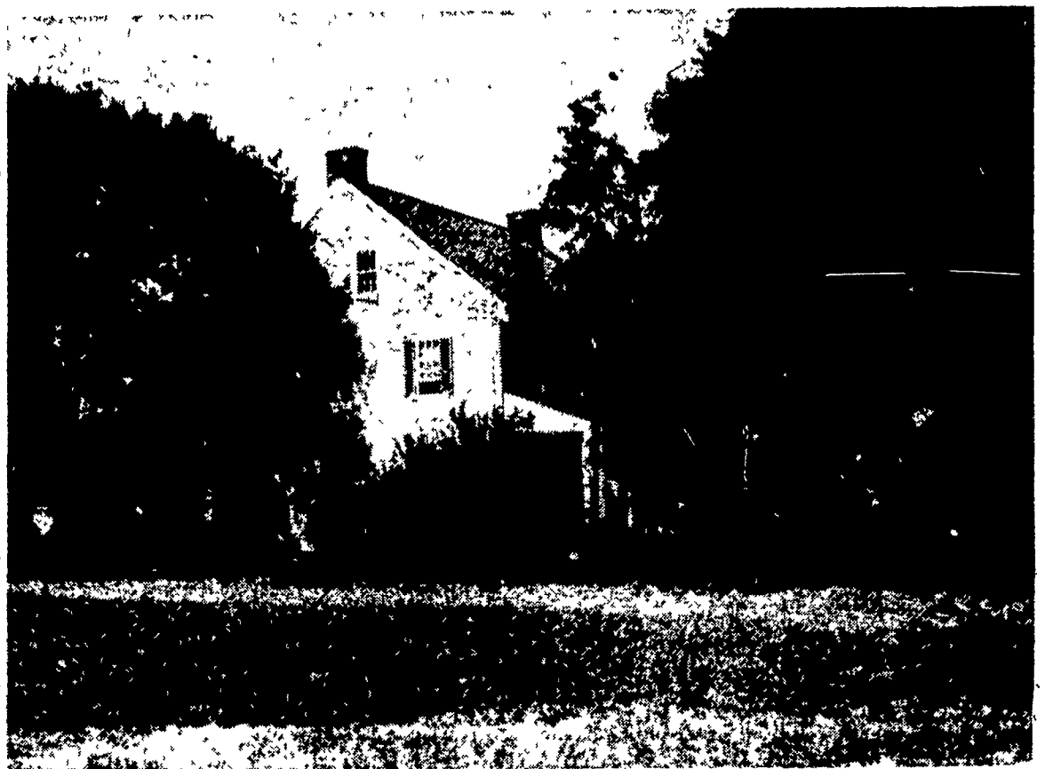
Now developing is the Pennsylvania State University Experiment Station at Landisville. On the right is the residence, which will be converted into offices, and
