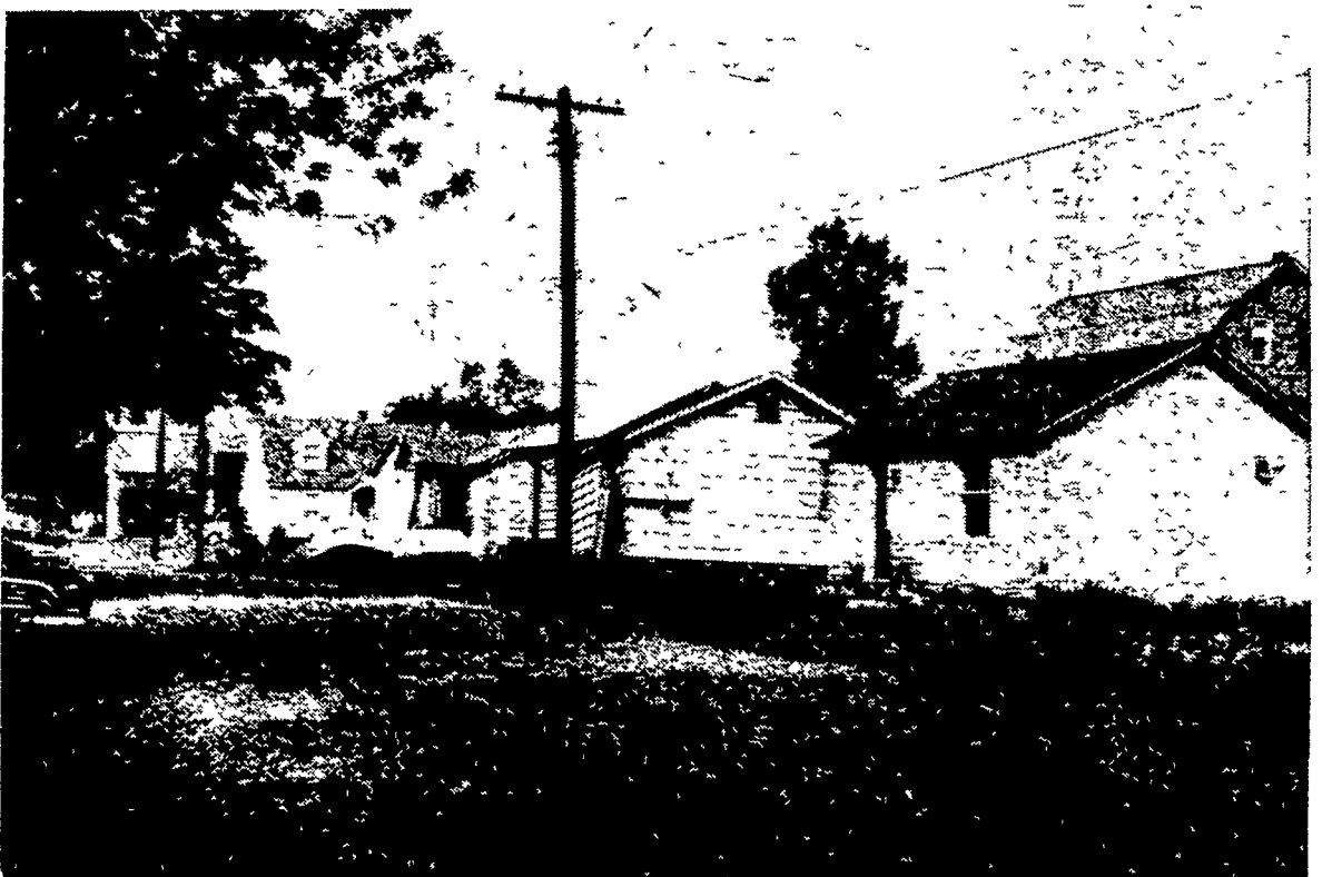
Streets have been resurfaced and many homes repaired or replaced in Stroudsburg. But for some, there was no opportunity or no desire to replace wrecked
