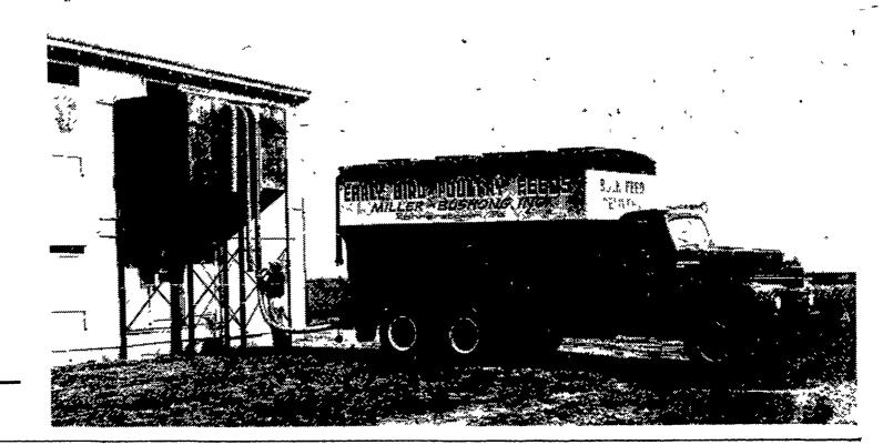
180 ton storage bins quickly load delivery truck for prompt delivery. A 45 ft. scale under bins preweighs feed at mill and assures you of accurate, full-weight measures.
