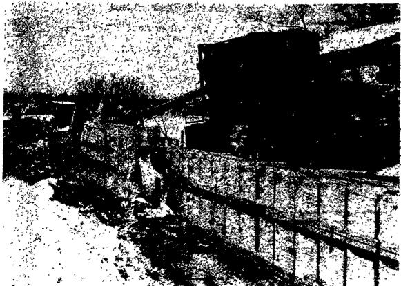
The weather was snowy, the ground was white, but nothing stopped the Sordoni Construction Co. when it was time to pour ready-mix concrete at the new Pennsylvania Community Telephone Co. Building in Quarryville. Luther Davis, construction superintendent, heads the crew. Here the east wall is starting to rise.
