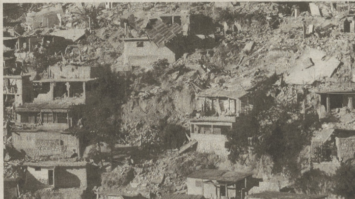
Debris on a hillside in Haiti. Photo courtesy of CNN.com.
