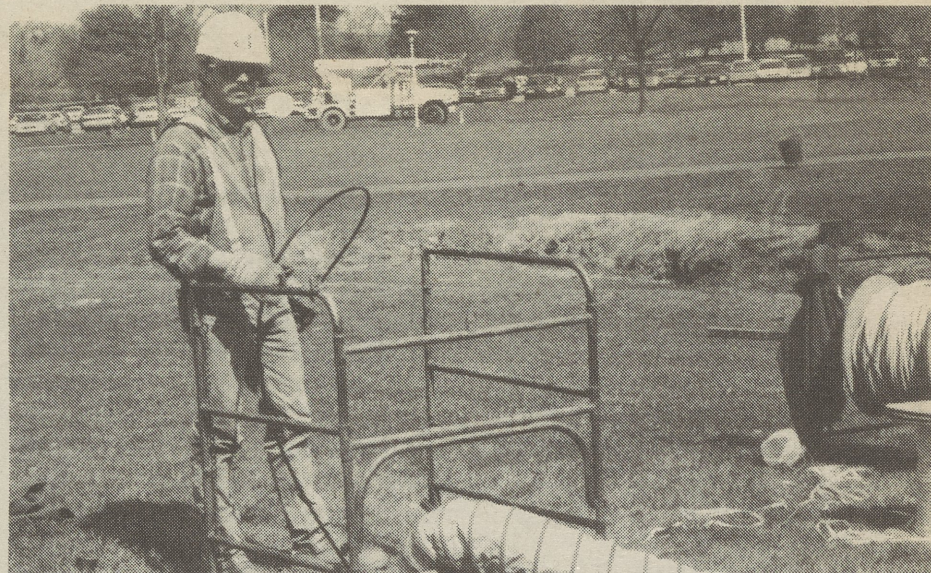
Fibreoptic cable being installed for future communications on Delco Campus.
