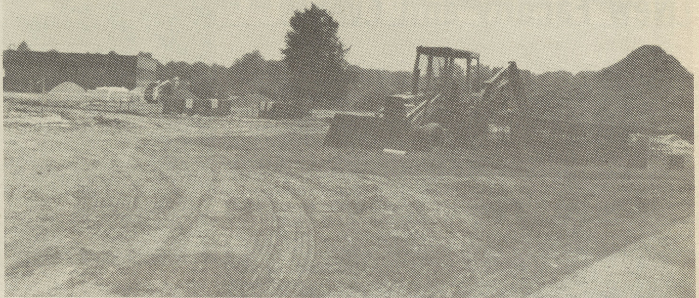
Construction for the new tennis courts begins.
