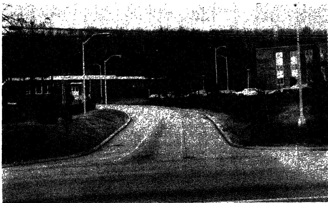
Work will soon begin on the Highacres Campus front entrance on Route 93. Lions and gates will make a more noticeable and attractive entryway.
