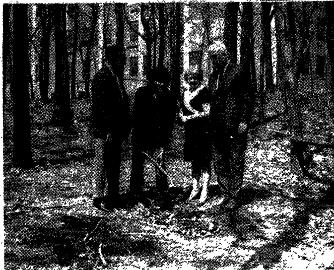
Groundbreaking for the Library
