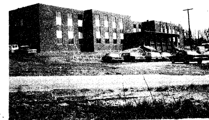
CO-ED RESIDENCE HALL presently under construction at Highacres will house 206 students.
