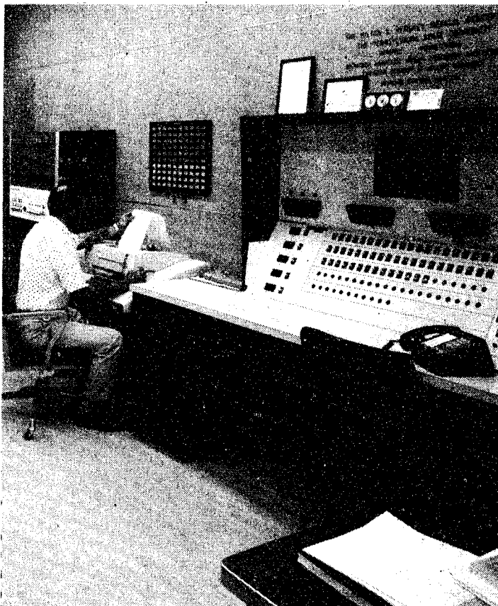
ONE MAN CAN MONITOR all mechanical systems of the Hospital and Medical Sciences Building of The Milton S. Hershey Medical Center of The Pennsylvania State University from this small room called the Building operations center.
