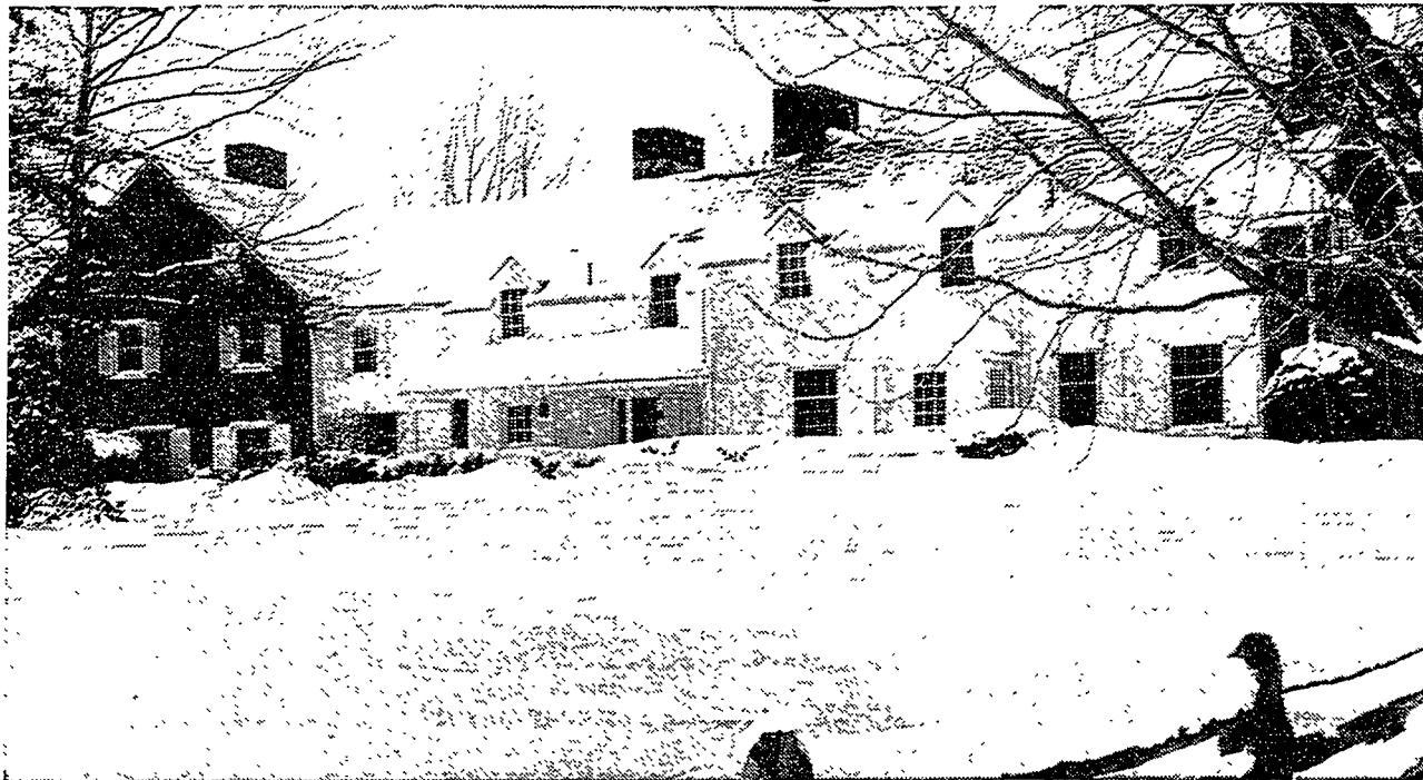
The Behrend Administration Building as it looks today, and much the same as it looked when occupied by the Behrend family.
