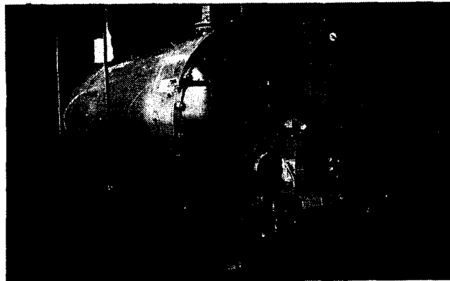
Contractors continue installation on the second of two new boilers. Workers cut a hole in the side of the heat plant structure (right) large enough to place the new equipment onto the second floor. Beautification on the heat plant building is pending.
