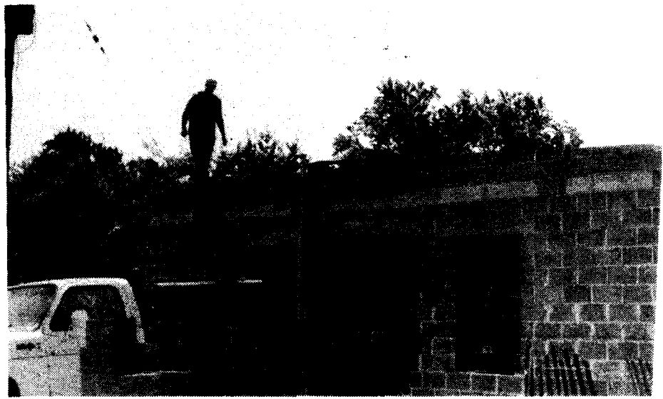
Admissions Building addition during the early stages in July.
